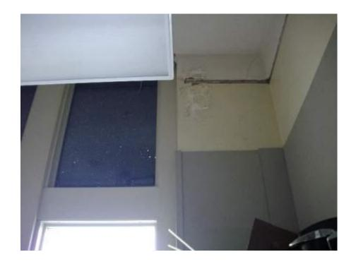
Typical window head on the third level. Water damage to window head and wall.
