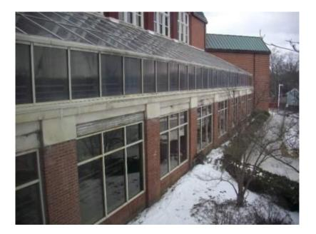
Hallway atrium in disrepair. Full re-build required in any renovation.
