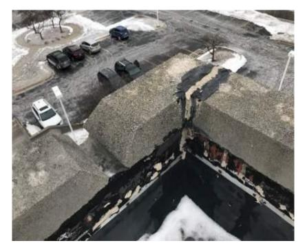
Typical issue for the top of the wall where there is stone coping. Roof membrane should go up the wall and under the stone coping.
