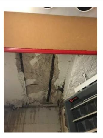
Room under exterior walkway. Damage has been caused by the infiltration of water and room should be demolished.
