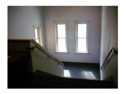
Stair to be enclosed and combustible material replaced. Under renovation, code dictates stairs to be enclosed.
