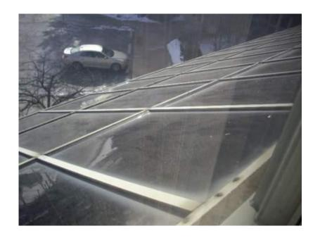
Typical condition of main corridor sloped skylight. Design does not allow for free flow of moisture.
